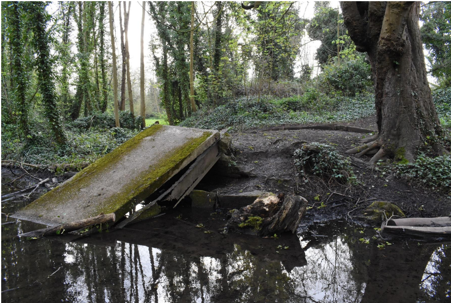
Plate 5: Side view of one of the surviving concrete floors with the metal beam remains underneath (facing E).
