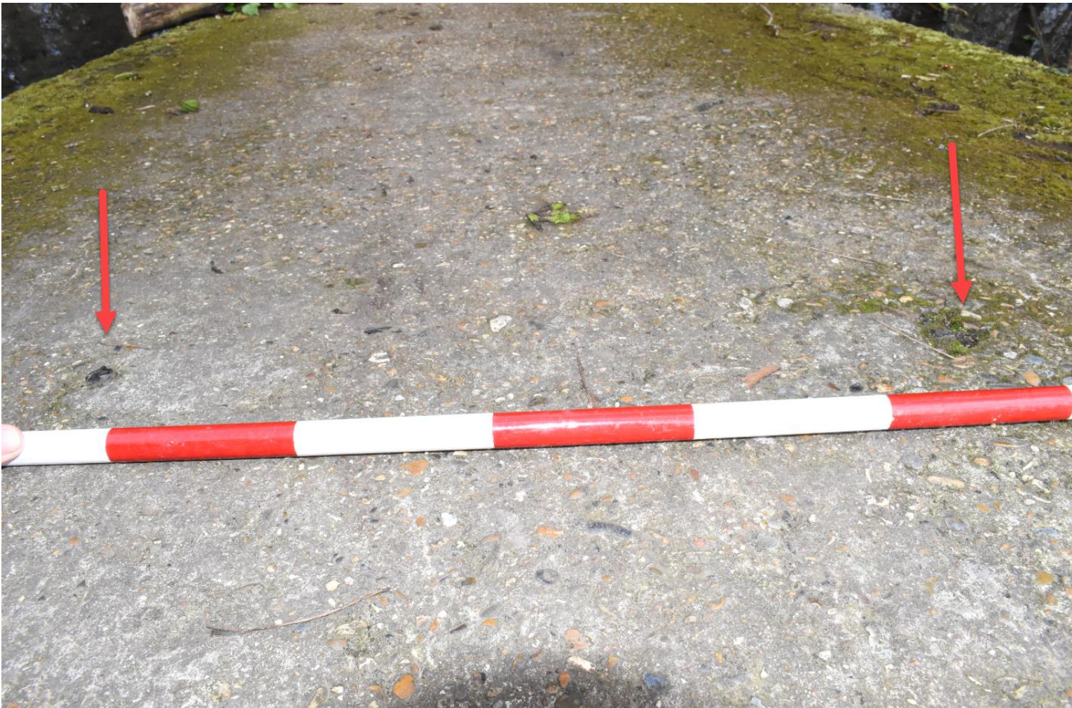
Plate 7: Showing evidence of the metal studs in the concrete floor, Scale 10cm intervals (facing NNW).
